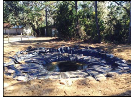
Dragonfly pond, newly excavated and lined with plastic, being filled with water. January, 2014
